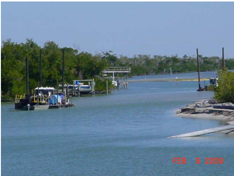
Monday, February 09, 2009 Dredging Operations in Wulfert Channel
