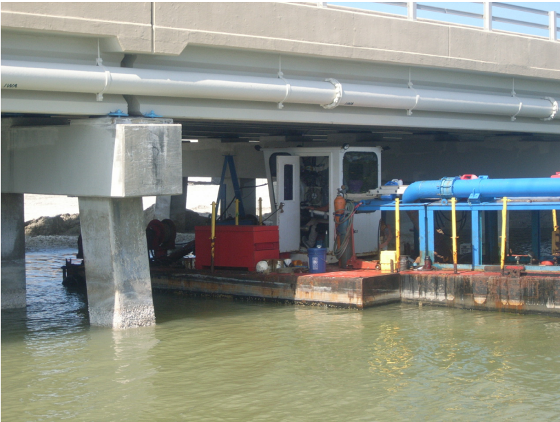
Thursday, April 16, 2009 Dredging Underneath Blind Pass Bridge
