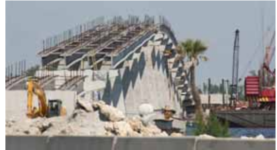
Bridge Photos taken by Rusty Isler on 9/24/06
